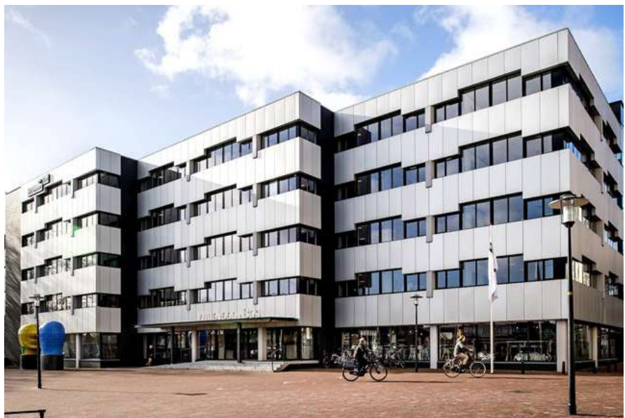
The offices of Witteveen+Bos in Deventer
